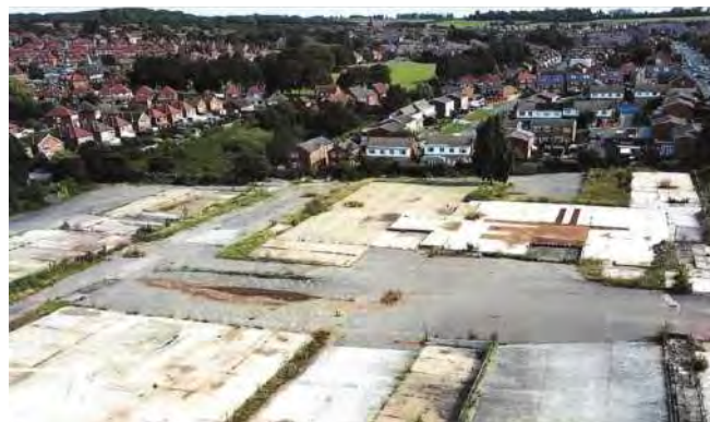
Figure 8: The site of our first ever modular build construction scheme in Arnold, Gedling.
