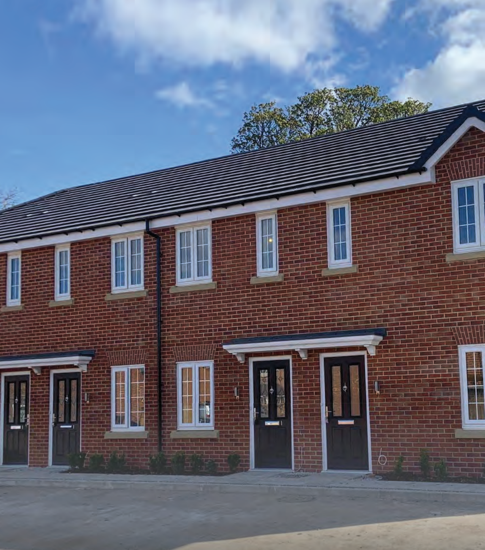
Calder View Catterall, Lancashire
