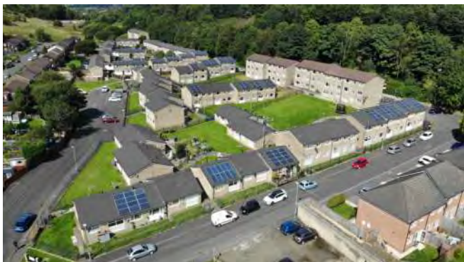
Figure 8: New energy efficient roofs with solar panels installed across homes in Waterton Lane, St Annes.
