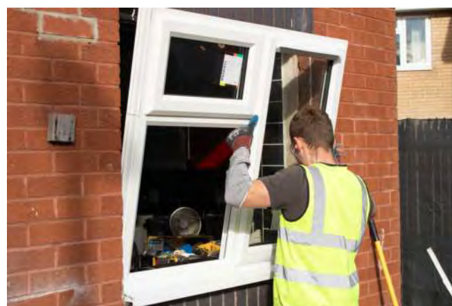
Figure 16: Improving thermal efficiency by replacing windows in homes across Tameside.
