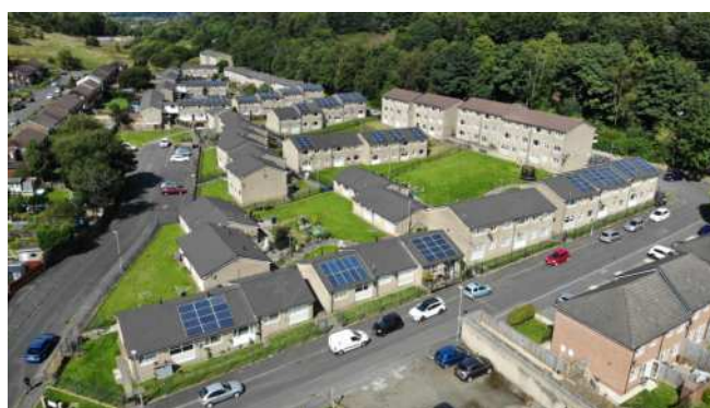
Figure 6: New energy efficient roofs with solar panels installed across homes in Waterton Lane, St Annes.
